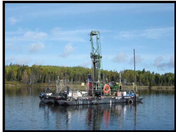
TBTE Drilling Barge
